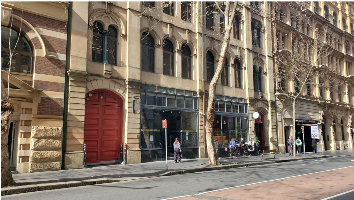
York Street frontage
